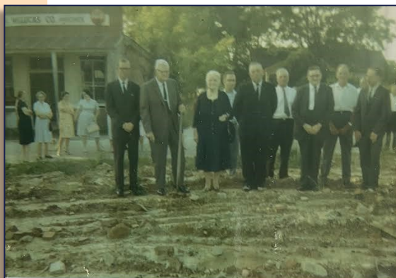
Ground-breaking for our new church (1965)
